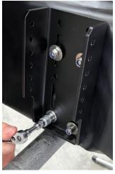
13. Feed four (4) M8 x 30 Hex Head Bolts (Item F2) through the hinge end of the awning and bag as shown.
