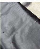
11. Cut another 10mm slit perpendicular to the last at each centre mark to form a cross slit.
