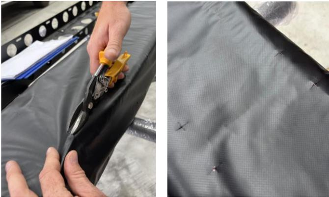
11. Cut another 10mm slit perpendicular to the last at each centre mark to form a cross slit.
